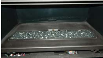
1) Start installing Crystals on the Burner
